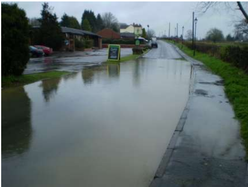
Coate Lane flooded by the Spotted Cow at Coate, March 2008
